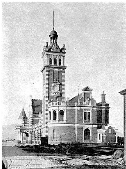
The new and imposing Dunedin station building nearing completion in 1906, as seen from the south end.
