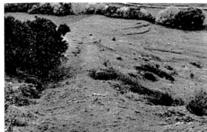
Photograph: P. F. Dyer, 1959 Looking down the site of the incline from the quarry towards the site of the sidings at the foot where trains were made up for haulage to Gisborne.
