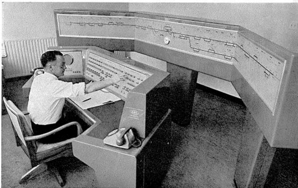
ABOVE: At Palmerston North, the push-button switches for the Otaki-Marton and Palmerston North-Woodville C.T.C. installations are desk-mounted, but the illuminated track diagram is erected separately.
