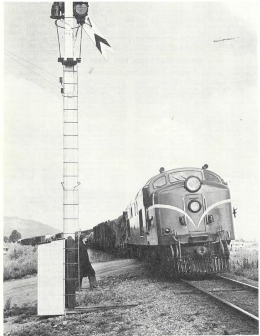
ABOVE: A "Df" class diesel-electric locomotive with a Wellington-Auckland goods train near Otaki in 1954. Note the large diameter of the main headlight as originally fitted.
