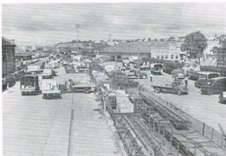
ABOVE: A busy scene in the Auckland goods yard in the 1950s.
