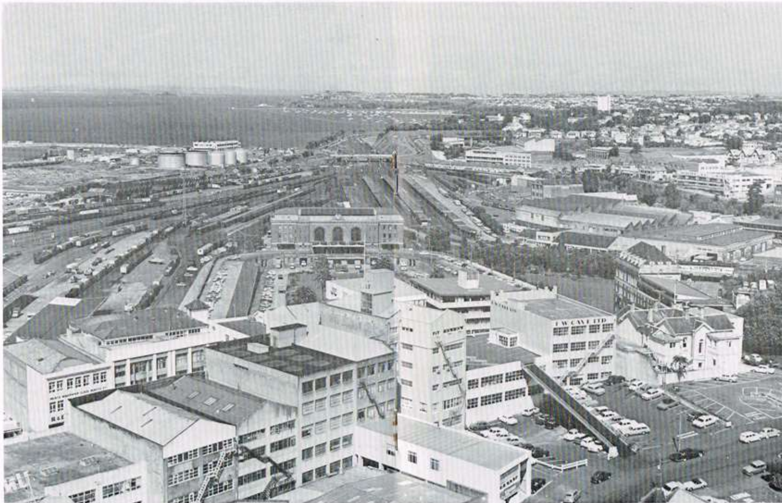
Auckland Railway Station and a section of the yards in the mid-1960s, looking from west to east. The platform tracks are numbered 1 to 7 from left to right, Nos. 2 to 7 being through lines.
